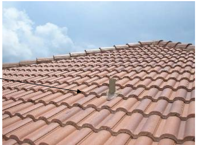
Location of the previous photo.
