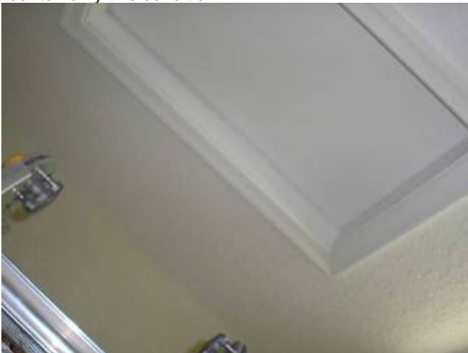
We were unable to verify all corrections in the attic as we were requested by the builder not to leave the ladder.
