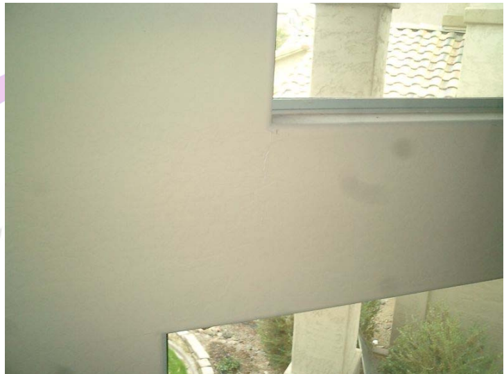
View of vertical crack and moisture stain at foyer wall between windows.
