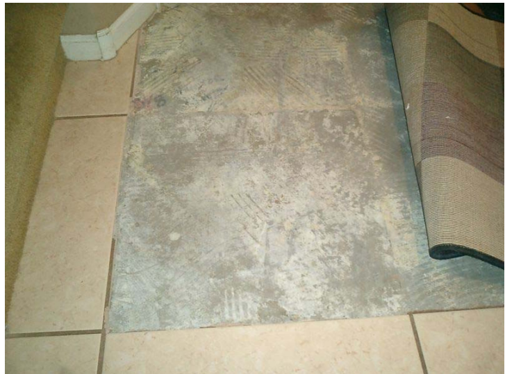
Close up of concrete in kitchen at base of stairs.
