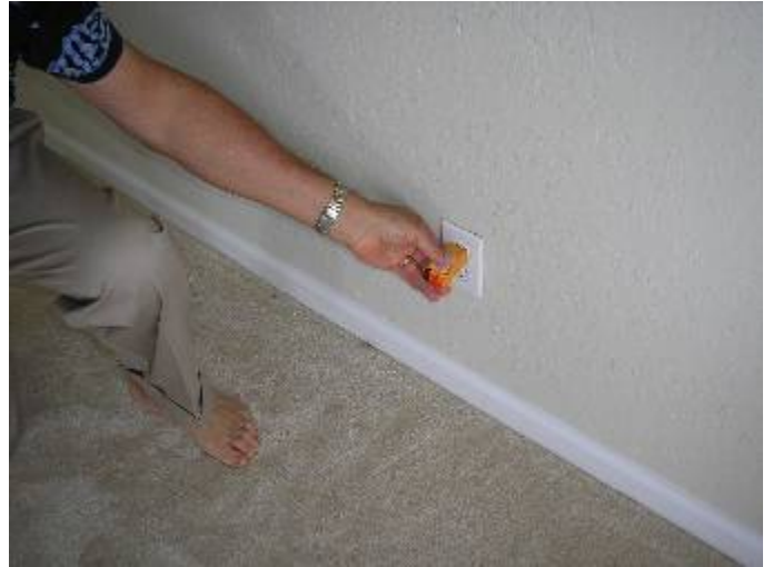
The outlets were loose in the wall after the repair was completed.
