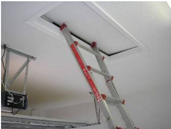
Location of the next photos taken from the attic access hatches.
