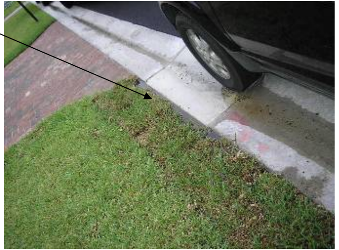
The sections of the front yard were very wet did not appear to be draining correctly.
