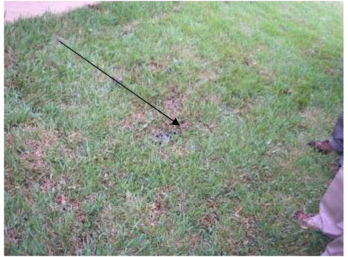
The yard at the sides of the building are very wet & did not appear to be draining correctly. The rear yard appears to be pitched towards the building.
