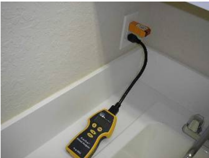
The laundry room receptacle outlet was repaired during the inspection.
