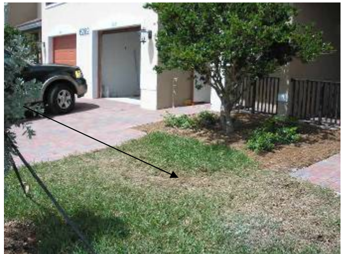
Some of the grass is brown &/or dying from what appears to be foot traffic at the front of the building.
