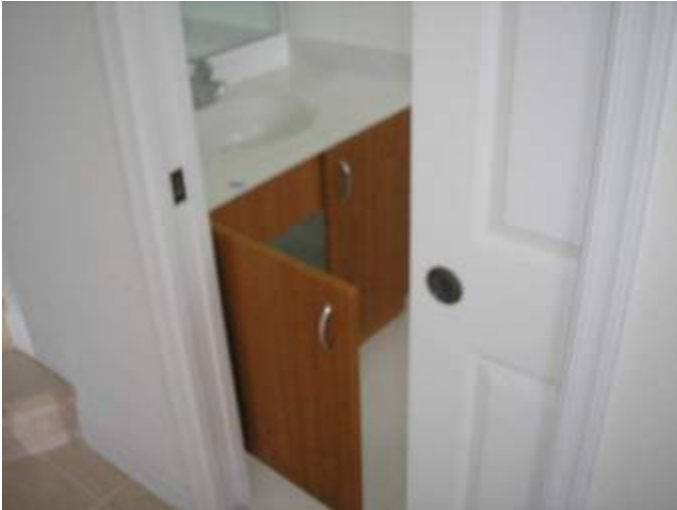
Location of the previous photo/s at the 1 st floor bathroom.
