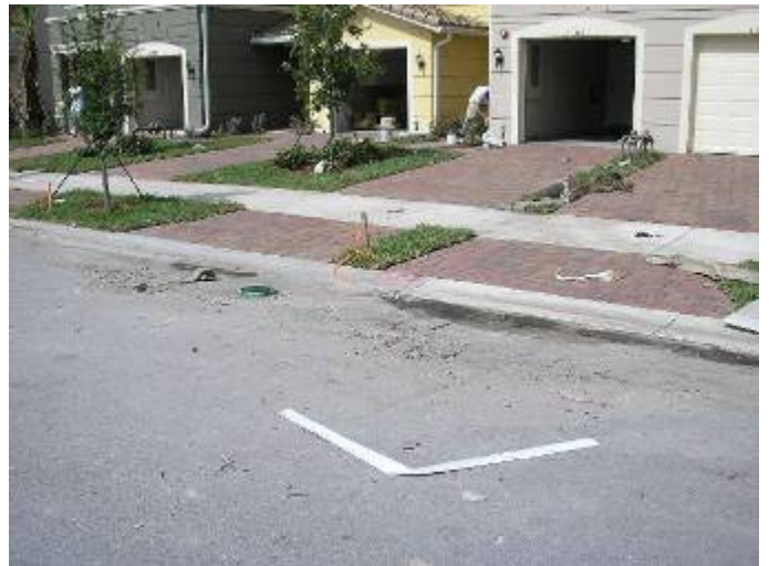
Trash & construction debris should be removed from the front of the house.
