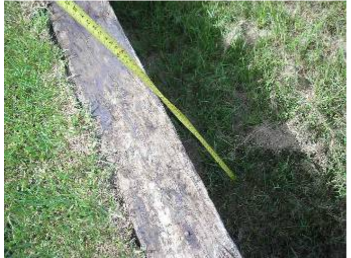
The railroad tie wall is almost 3 feet high, has no railing & presents a tripping/safety hazard at the back of the building. FBC §1617.4.4
