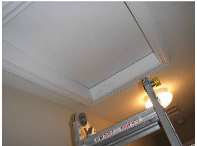
Attic inspection begins.
