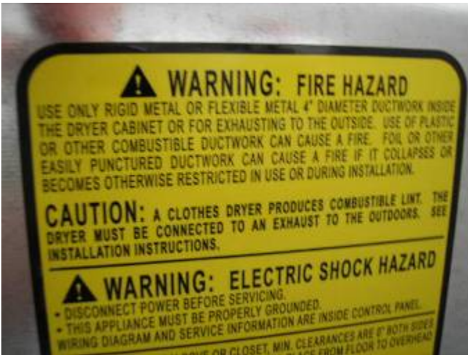
The thin aluminum foil dryer vent duct material is a fire hazard per UL & manufacturer. See warning label on back of the dryer. §M304.1
