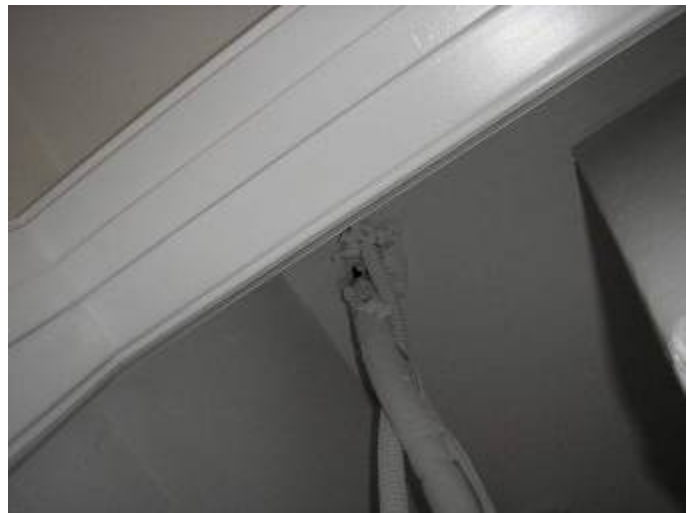
The AC mechanical closets are not completely sealed as required. The air handlers have not yet been installed.
