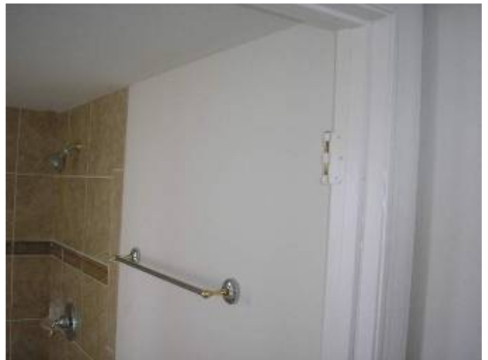
Some of the interior doors were not yet installed.
