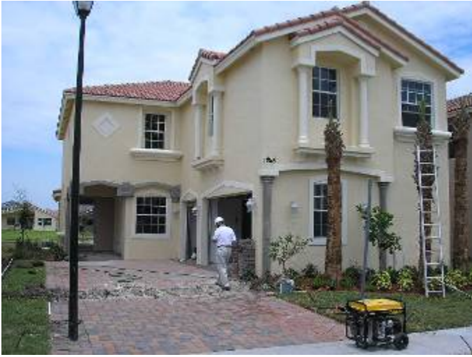
Site photo. The front of the house faces towards the east.
