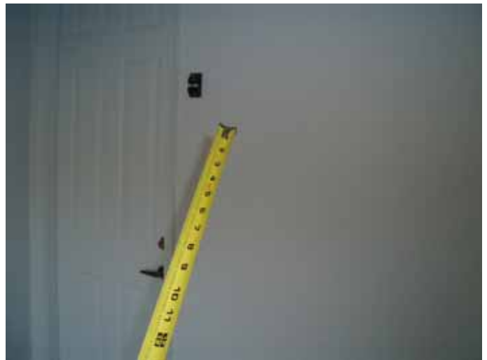
A warning label needs to go on the wall by the auto door opener switch §M304.1
