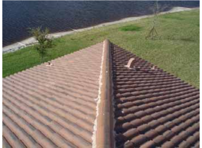
Location of the previous photos.
