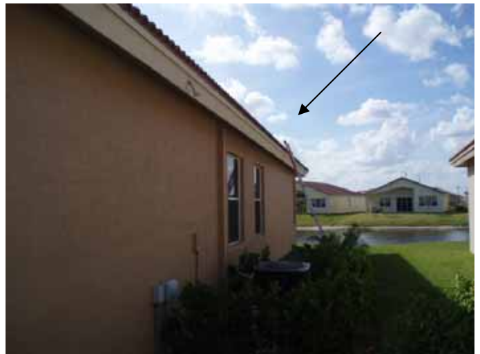
Location of the previous photos at the north side of the house.
