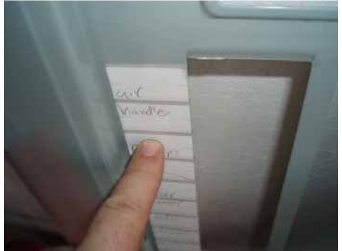
There were no electric heat strips located inside the furnace. The approved plans for this house should be reviewed & electric heat strips installed if required.
