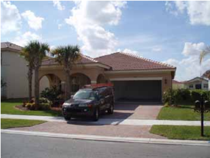
Site photo. The front of the house faces towards the southeast.
