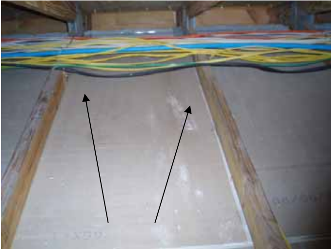
Location of the previous photos over the garage.
