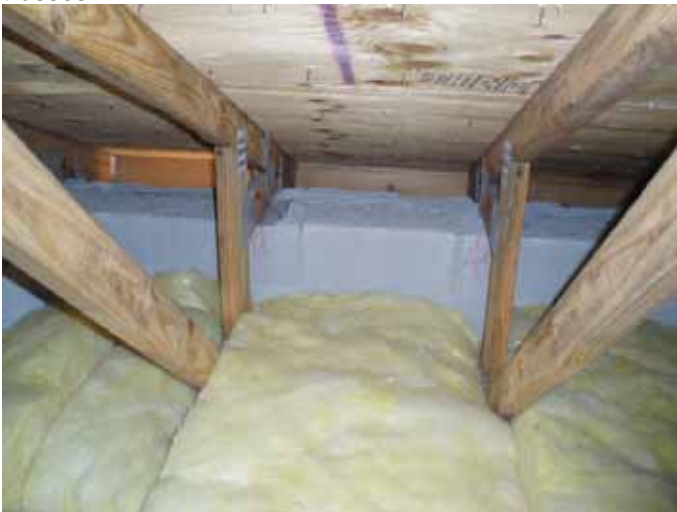
Location of the previous photos over the living room area.
