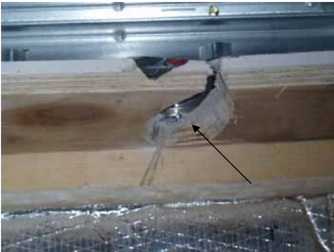
The AC make-up air (from the exterior) should be filtered.
