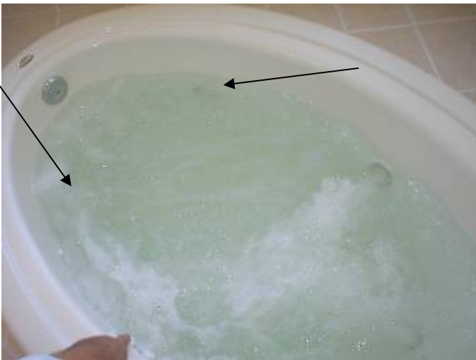
The front jets did not operate correctly at the whirlpool tub in the master bathroom.
