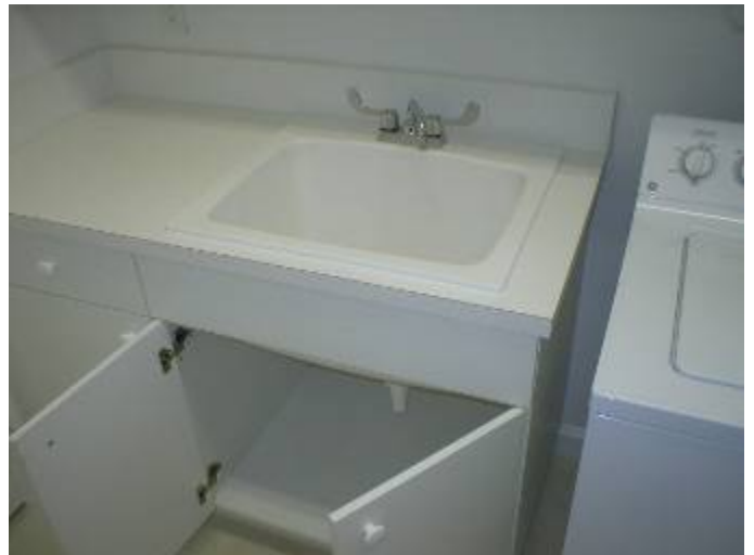
There are leaks at the plumbing drain line under the laundry room mud sink.
