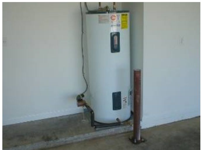
Location in garage.
