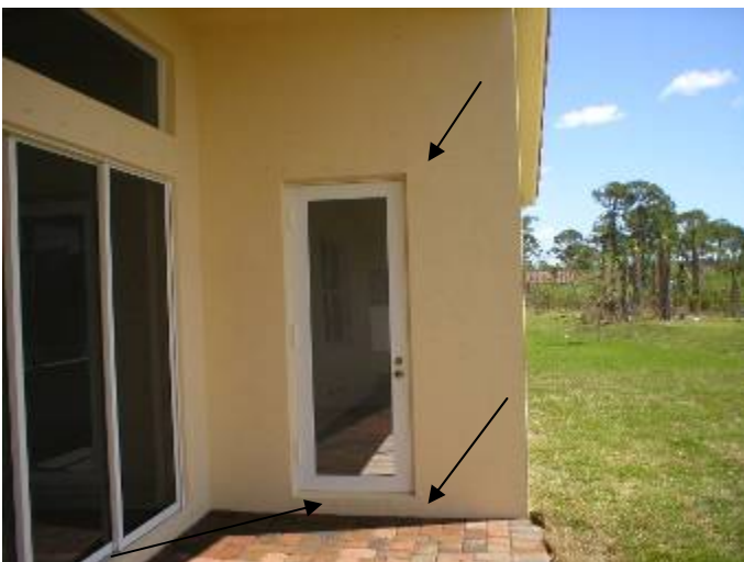
Location of the previous photos at the back patio.
