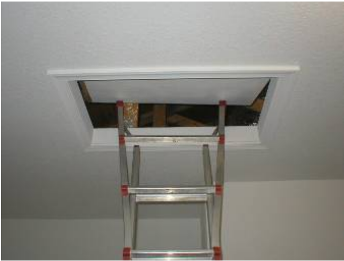
Next photos of the attic.
