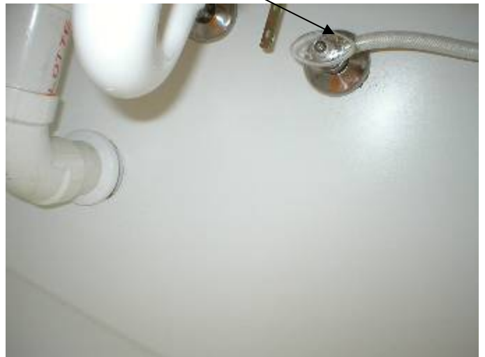
There are gaps & unprofessional looking cut outs at the back of the sink cabinets.
