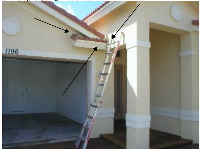
Location of the previous photos above the front of the garage. §1403.1.3 Veneered walls shall provide weather protection for the building at the walls.
