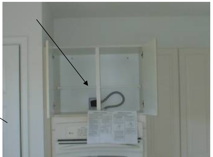
Location of the previous photo in the kitchen above the ovens.
