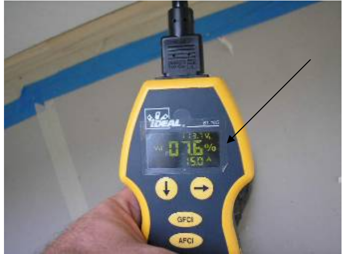
Many of the receptacle outlets had excessive voltage drops at the throughout the house. 2002(NEC) 210.19 Conductors
