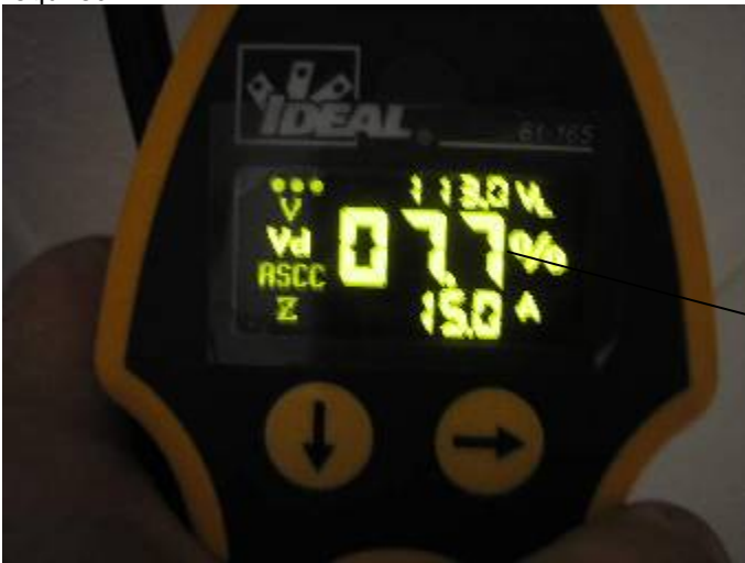
Many of the receptacle outlets had excessive voltage drops at the throughout the house. 2002(NEC) 210.19 Conductors
