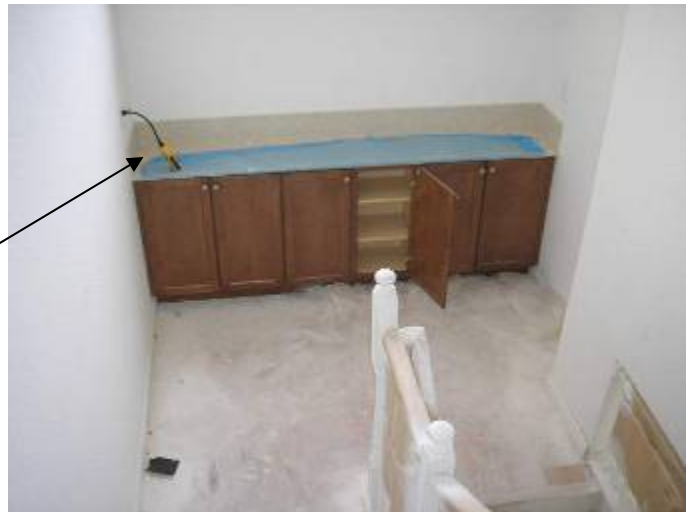
Location of the previous photos. The voltage drops should not exceed 5%. 2002(NEC) 210.19 Conductors
