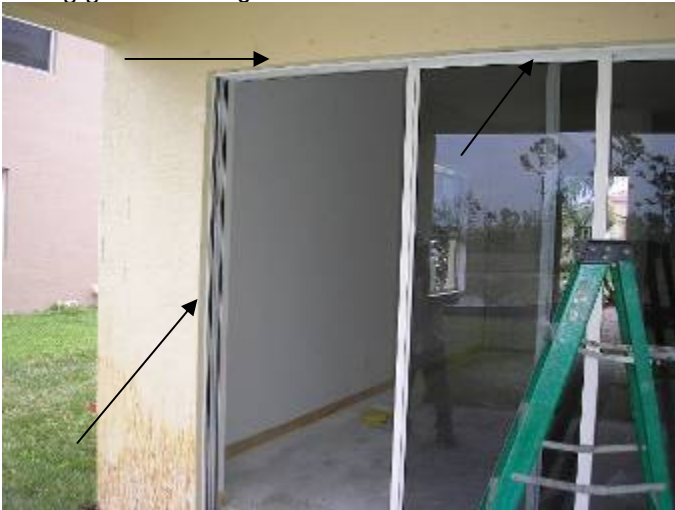
Location of the previous photos at the sliding glass doors.
