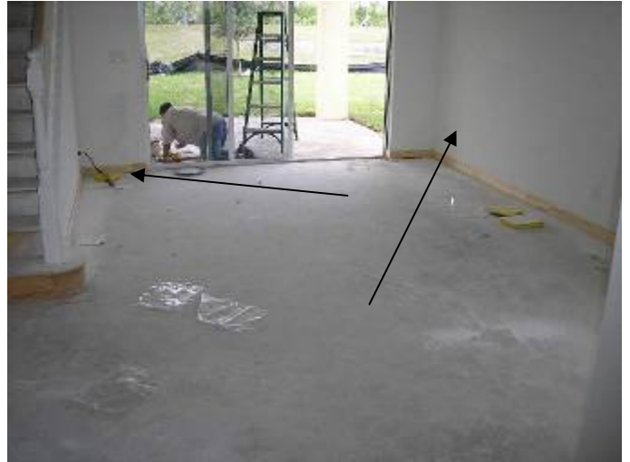
Location of the previous photos. The voltage drops should not exceed 5%. 2002(NEC) 210.19 Conductors
