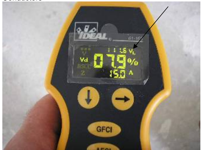
Many of the receptacle outlets had excessive voltage drops at the throughout the house. 2002(NEC) 210.19 Conductors
