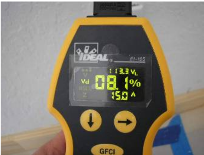
Many of the receptacle outlets had excessive voltage drops at the throughout the house. 2002(NEC) 210.19 Conductors
