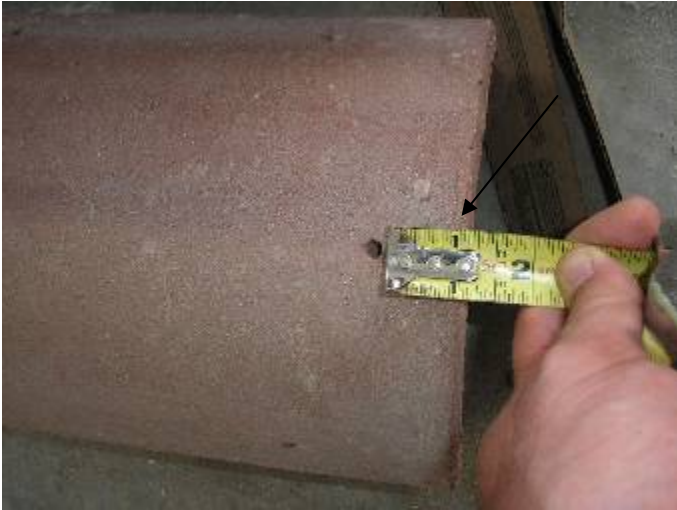
The openings in the ridge cap tiles measure approximately 1 inch from the edge. There should be no exposed nail openings in the tiles on the roof. §1518.8.11
