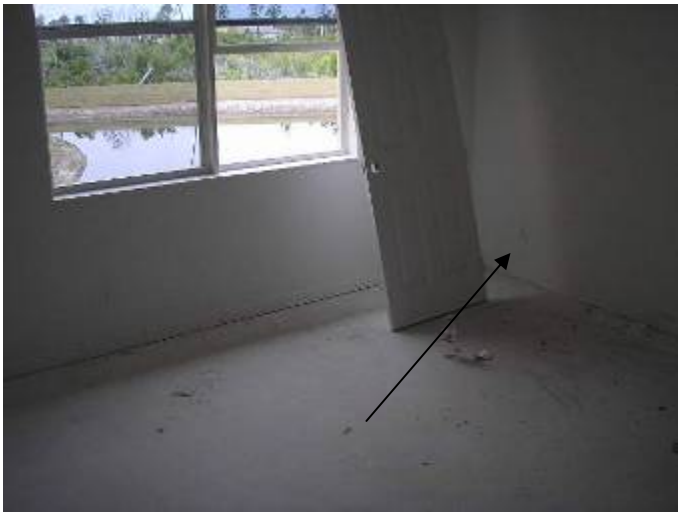
Location of the previous photos. The voltage drops should not exceed 5%. 2002(NEC) 210.19 Conductors
